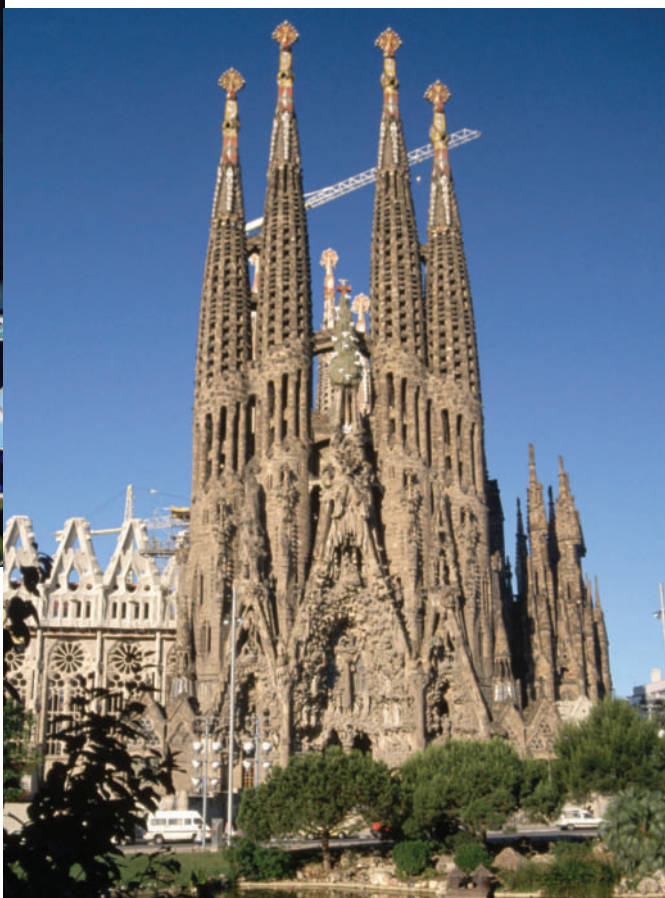
High ideals: construction work on Barcelona’s Sagrada Família church.
